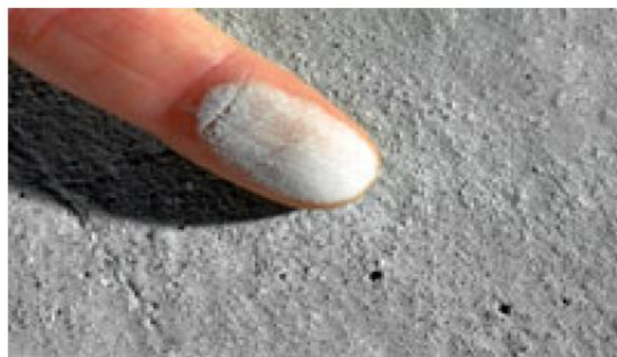
Fig. 3.11: Dusting of Concrete Surface. ( http://www.prairie.com )
