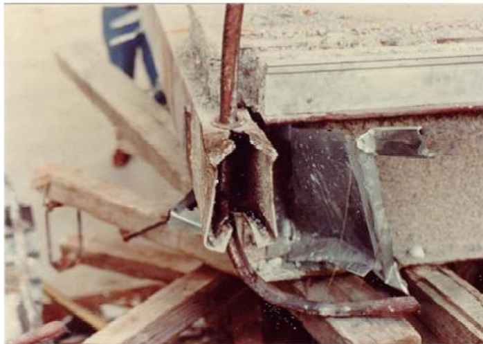
Fig. 6.2: Photo of one of the walkway cross-beam [4] .
